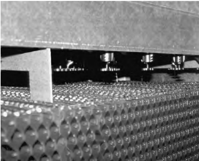
Eliminator air-seal removed showing nozzle distribution area above fill
